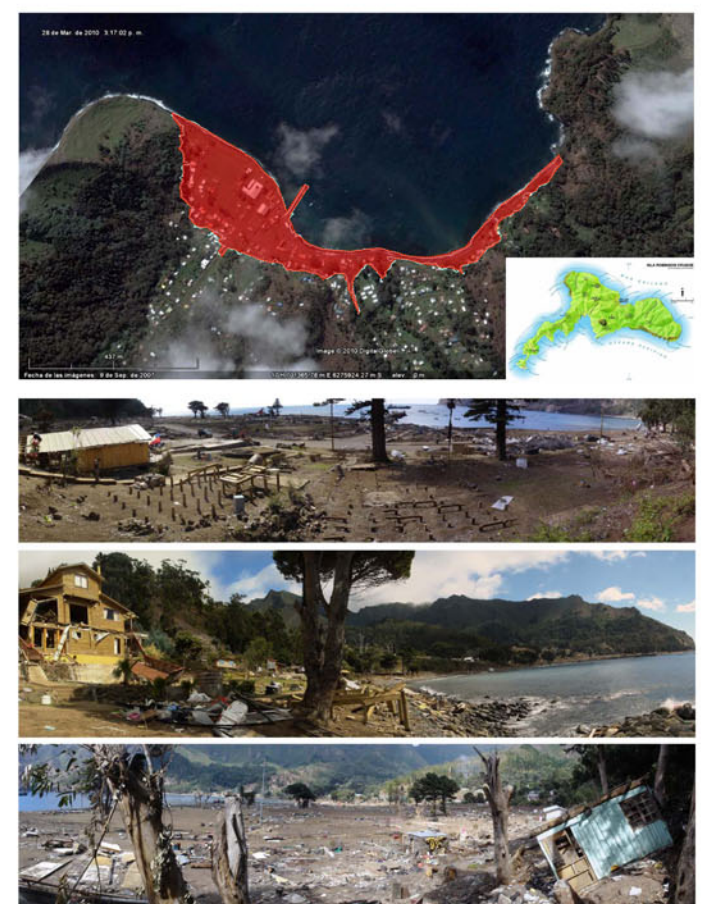
Figure 6. Archipelago Juan Fernández: (a) Mapped inundation at San Juan Bautista, (b) Destruction along Cumberland Bay (credit: Patricio Winckler, Universidad de Valparaíso, Chile).
